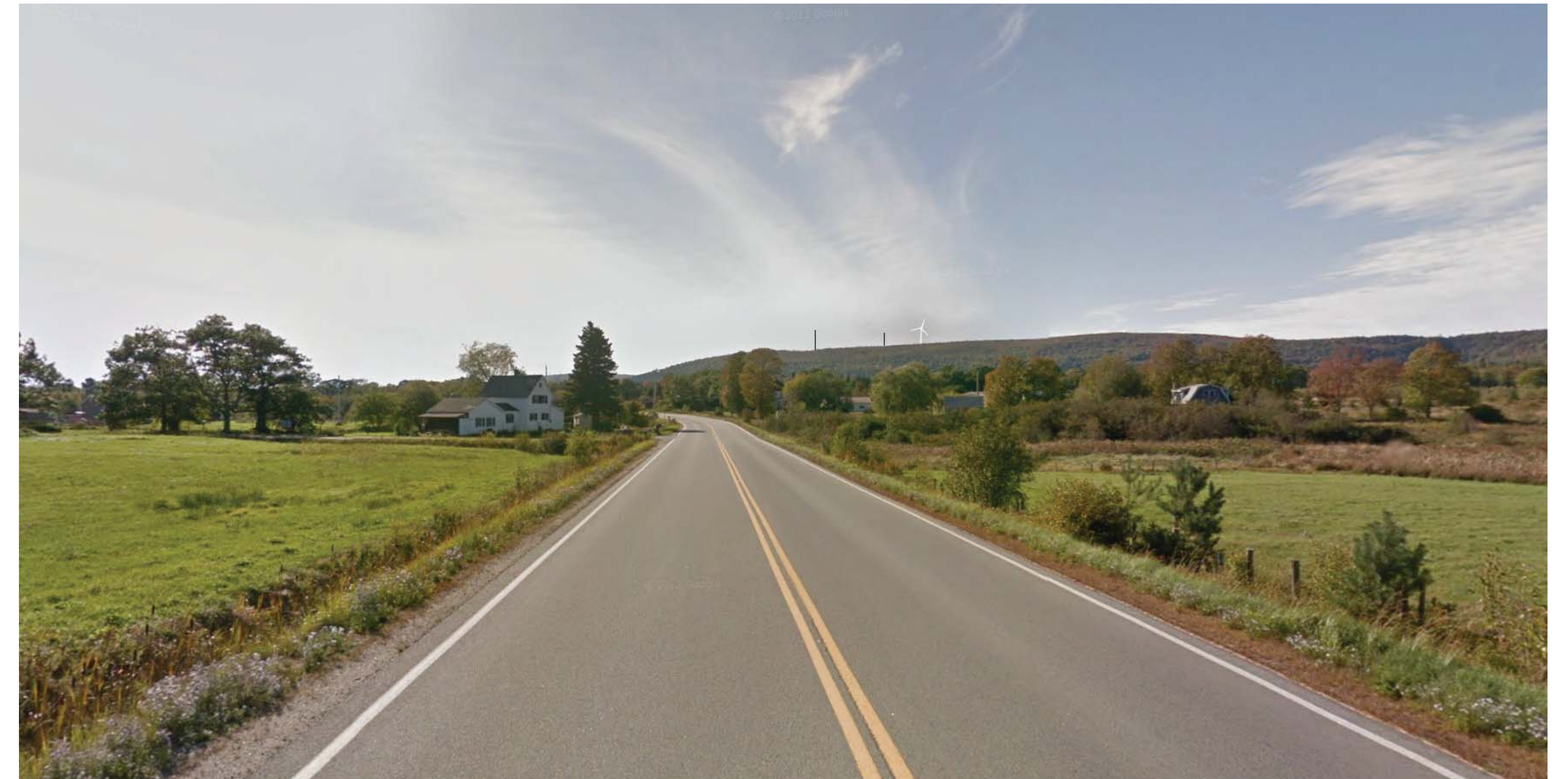
View 4 - Evangeline Trail at Granville Centre: Looking West
